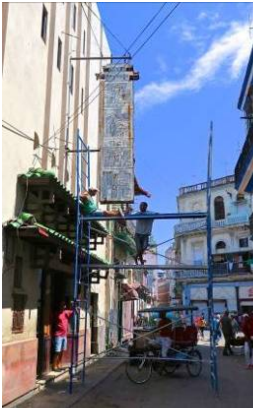
GALLERIA CONTINUA / Habana Entrance to the gallery in the Chinese district of Havana. Work in progress
